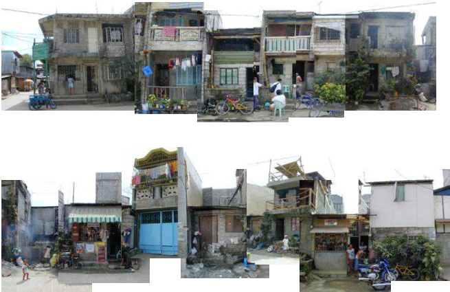
Figure 2. RC Frame with Masonry Wall Structure in the Resettlement Site of Marikina
