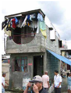
Figure 5. Existing House E
