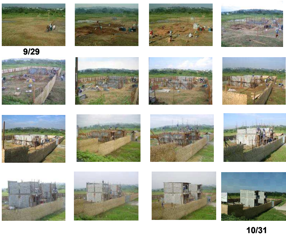
Figure 7. Construction of House N1 and N2 with Current Construction Method
