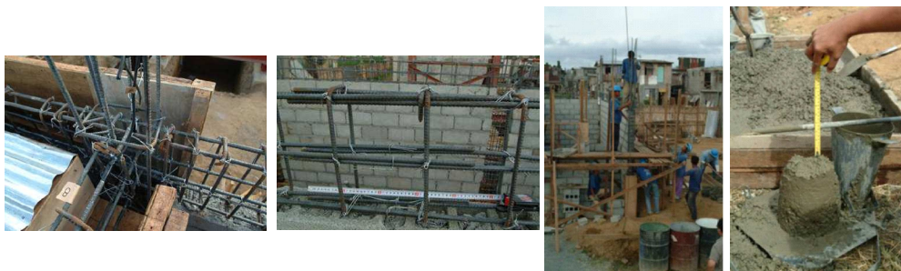
Figure 12. Construction Process for House R
